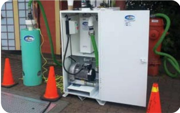
DO<sub>2</sub>E Little John Grease Digester Systems are designed for the treatment, control and removal of Fats, Oils, and Greases (F.O.G.). Little John Digesters eliminate grease build up and matting, reduce H<sub>2</sub>S levels, and help control ragging problems at sewage pump stations and grease interceptors.
